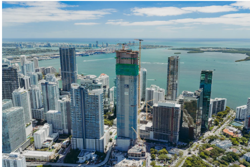
The Cipriani Residences Miami is under construction. | Cipriani Residences Miami
